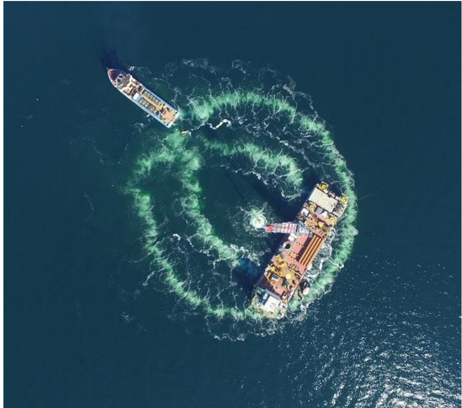
Figure 14.1: Example of active bubble curtain (double Big Bubble Curtain) deployed around the jack-up platform used for pile driving. Air bubbles are visible in the surface as the white ring. The ship in the front is used for deployment and retrieval of the hose system and contains the very large compressors needed to feed the bubble curtain with compressed air. Hydrotechnik Lübeck.
